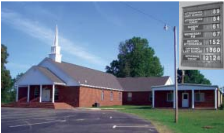
Newly Rebuilt Auditorium of the Antioch Church of Christ, near Tupelo, MS
