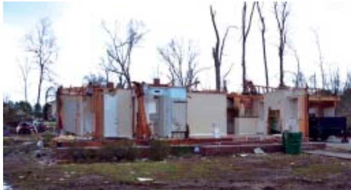
Tremendous Damage But No Lives Lost!
